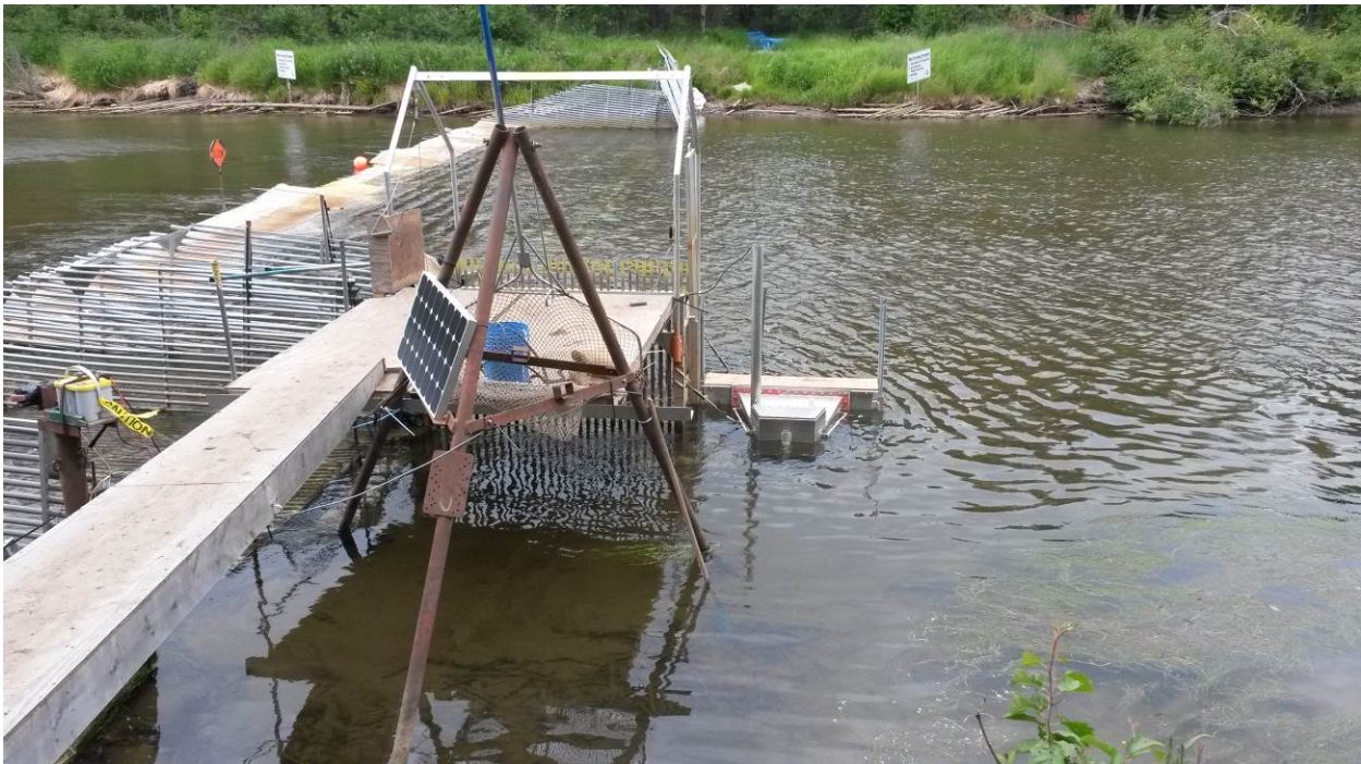
The completed Little Sustina River weir.
