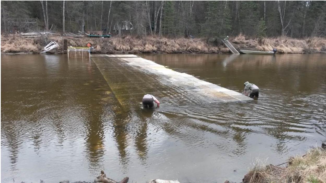
Weir installation at the Little Susitna River.
